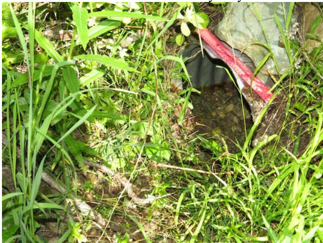
8378: (C) 18" culvert, currently dry.
