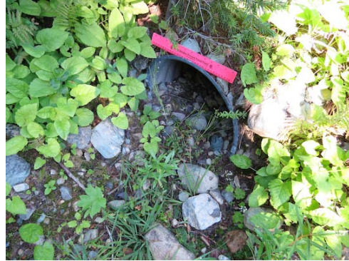
8375: 18" culvert inlet shown in 8374, one-third full of debris.
